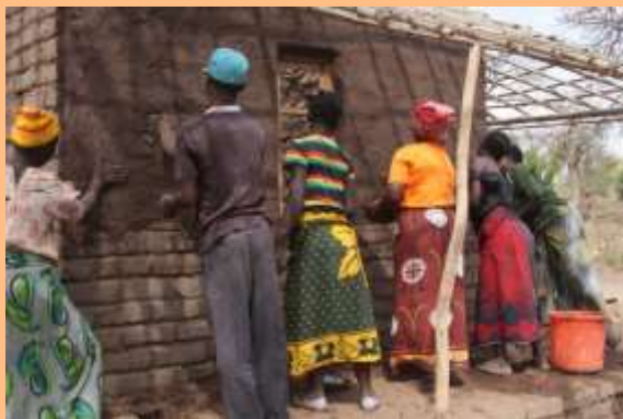
Walls are rendered using traditional techniques.
