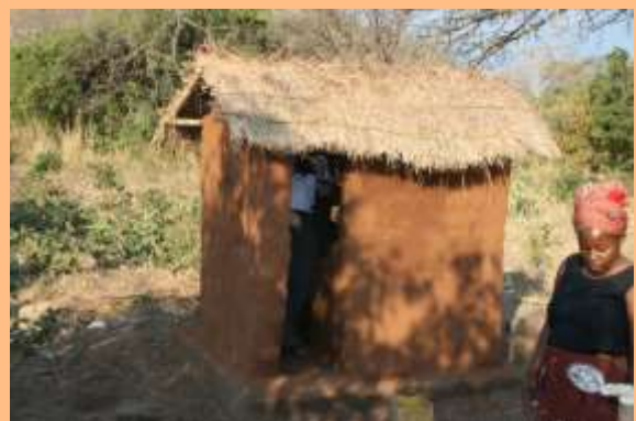
Latrine constructed by householder.
