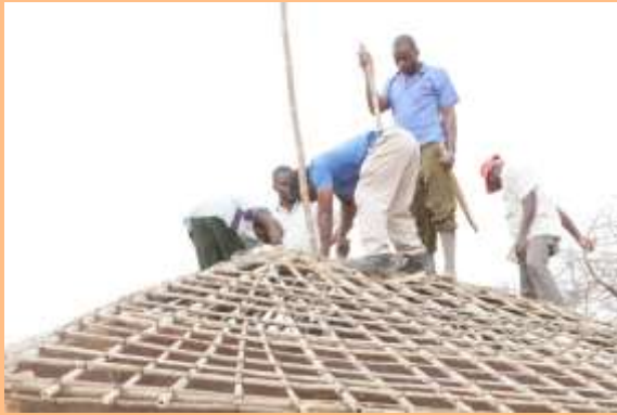
Rafters and battens fixed with tie wire. Wall plates fixed securely to posts and walls.
