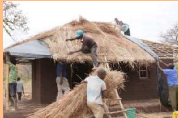
Thatch fitted over the membrane.
