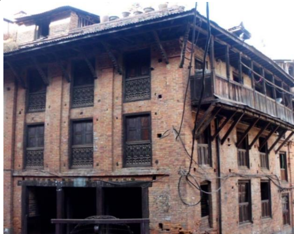
Fig. 1 Symmetrical matchbox construction practice at Bhaktapur
