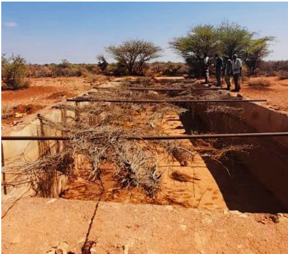
Empty berked in Bursalah, Mudug (Photo by SDC)
