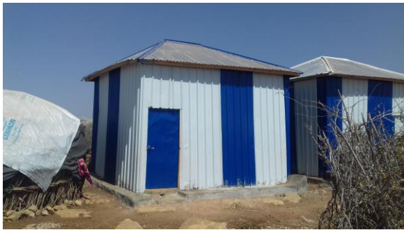
Transitional shelters constructed by returnees in Baidoa through cash enabled owner driven approach provided by INTERSOS / UNHCR. Picture by INTERSOS Baidoa.
