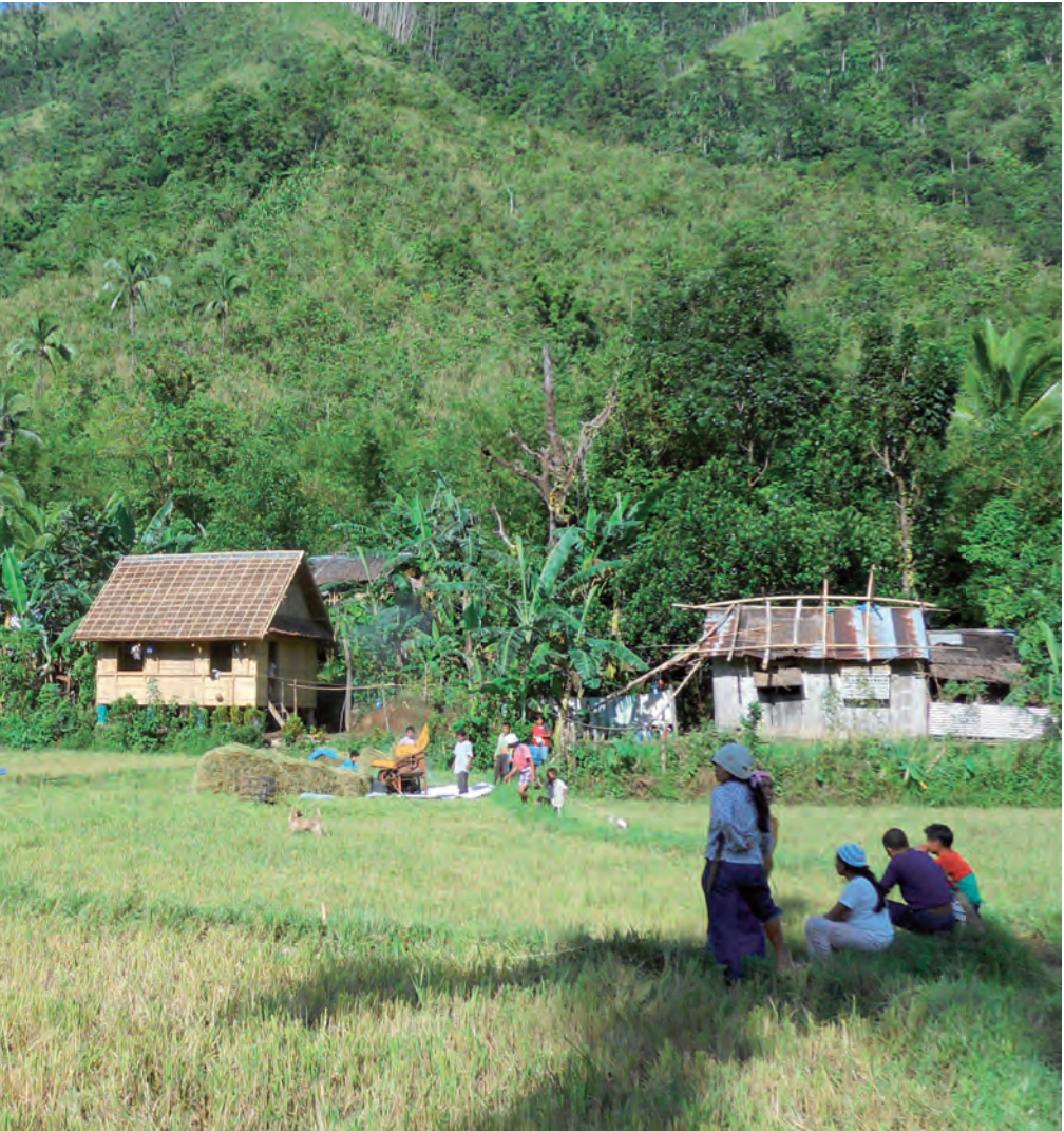
Philippines: existing house (right) and houses rebuilt after 2013 typhoon Haiyan with improved local techniques and materials (left)
