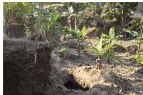
6. Soil erosion due to brickmaking
