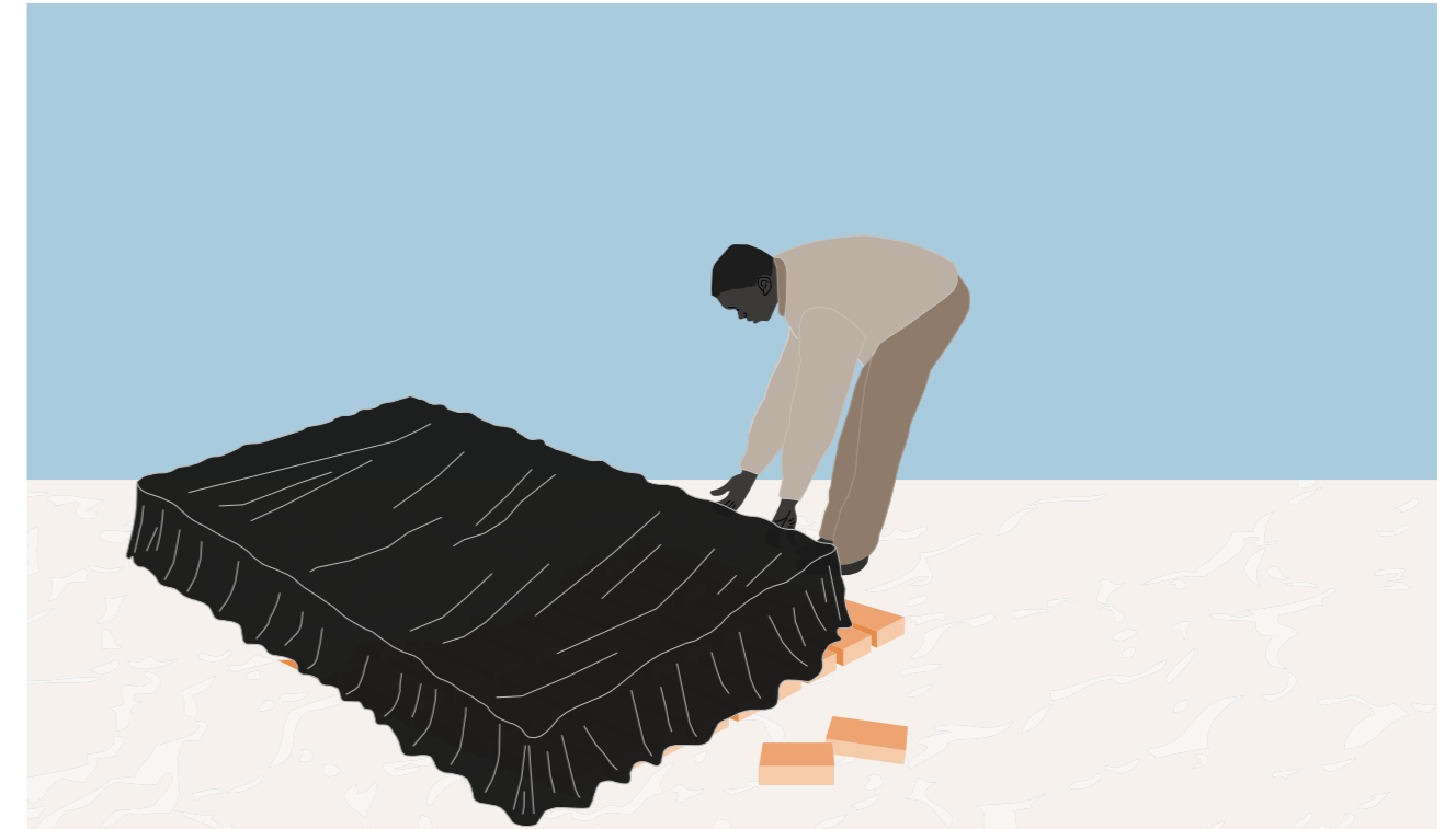
22. SSBs CURING UNDER PLASTIC SHEETS
