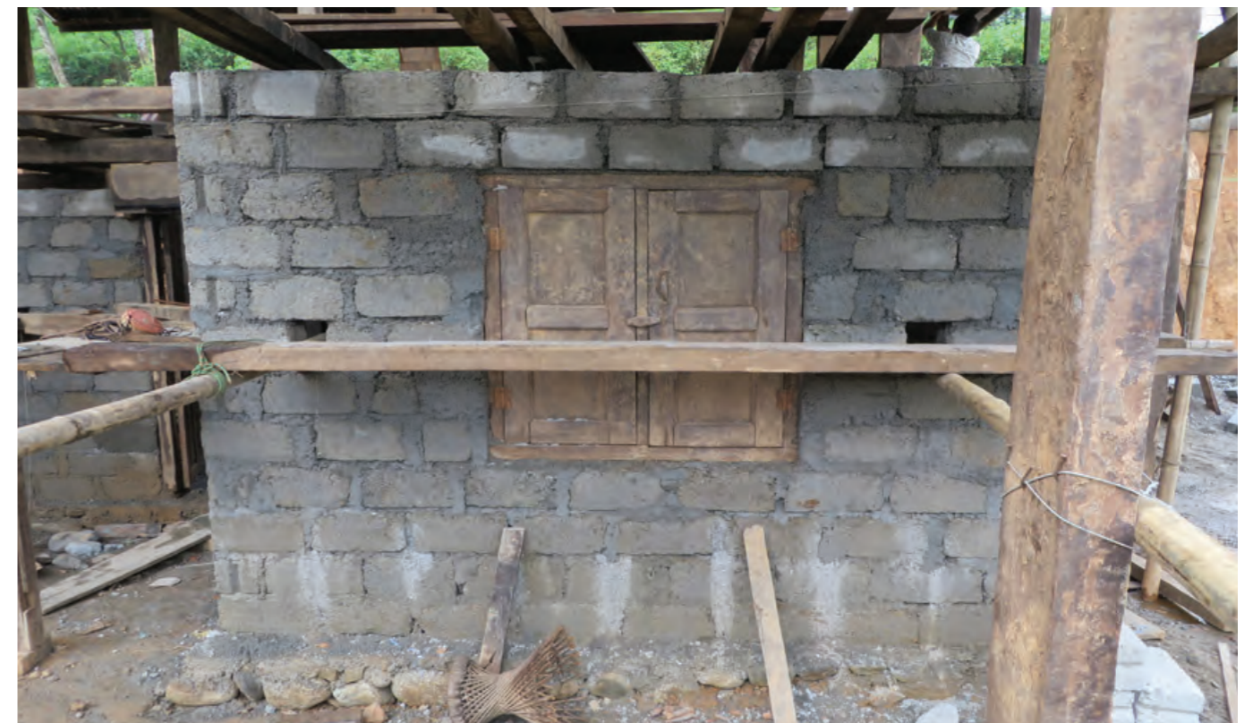
Sindhuli District, new concrete block construction replacing stone, June 2015
