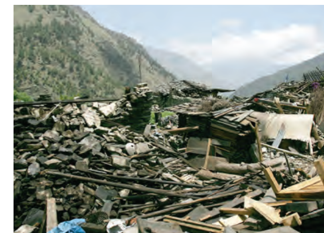
Earthquake damage, rural village.
