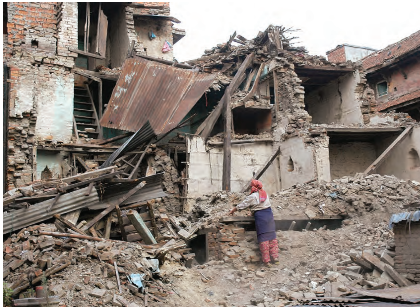
Bhaktapur, damaged homes in the old city, June 2015
