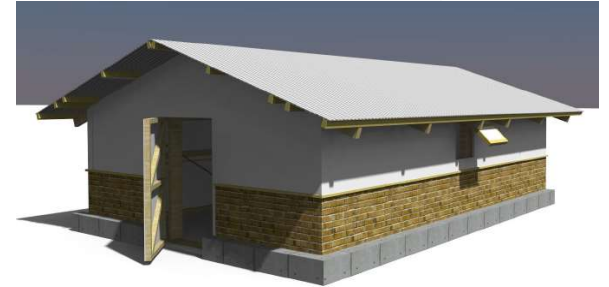
PHASE 3 Replacing the Tarpaulin wall at low height with low height mud brick and plaster
