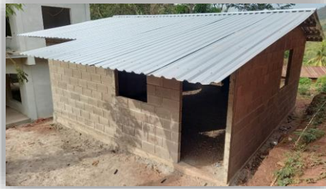
Roof and floor
