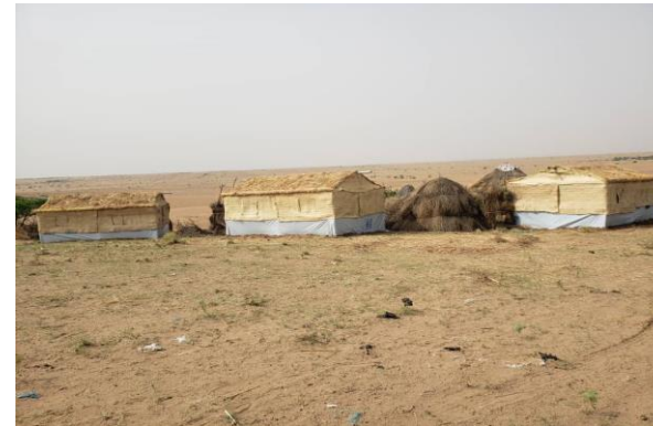
UNHCR/JAAH constructed 1310 TESKs for IDPs As Sukhnah district within AI Hudaydah.
