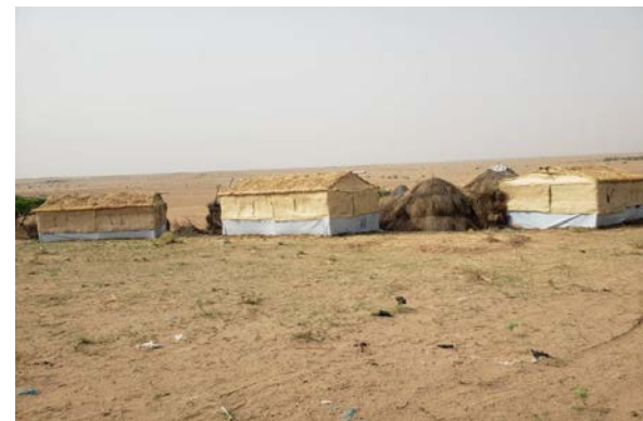
By YHPF funds, NRC team distributed cash for shelter maintainance for 500 households who their shelters are affected by heavy rain or environment conditions in Abs district within Hajjah.
