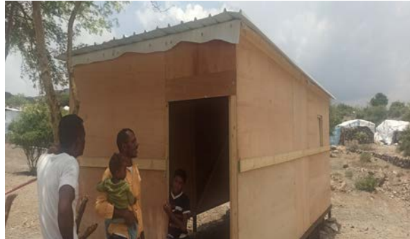
Transitional Shelters in the IDP sites in Al Ma'afer and Ash Shamaytayn districts implemented by IOM
