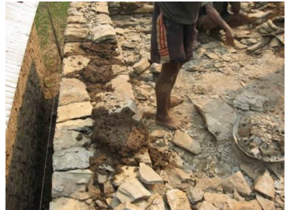
Photos by Prem K. Khatri of school construction in Gorkha district.
