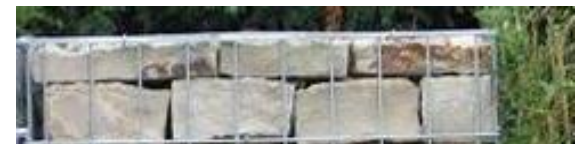
Photos from web of gabion basket retaining wall (above). The photo below shows how inconspicuous the wires can be if the basketing is of only a single layer of stone.
