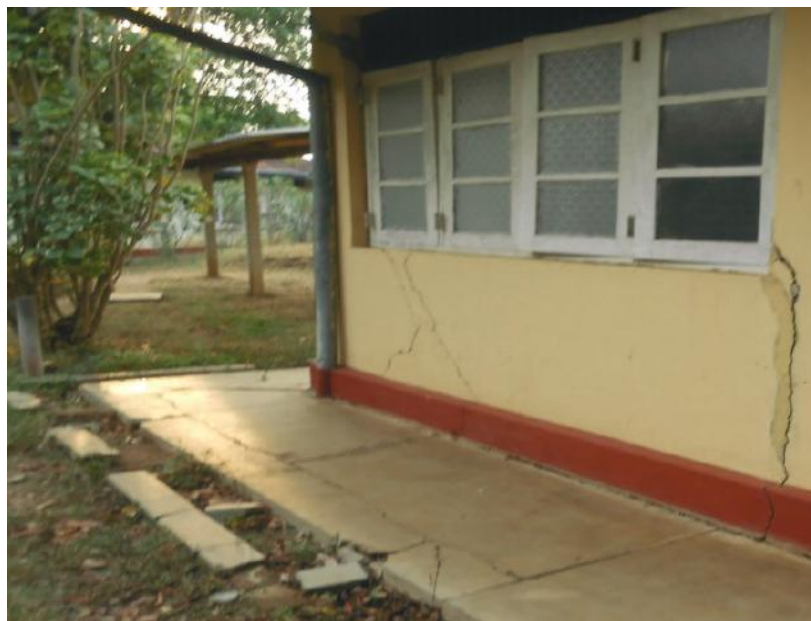
Image: 1b. Cracks on the Floor and Window Sills
