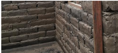
Adobe Blocks- Under construction (! rainy season)
