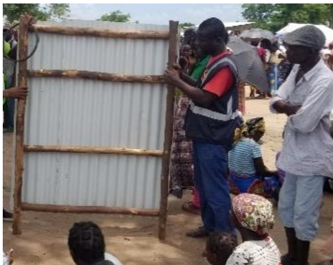
Training at distribution point- Fixing of CGI to pole roof structure
