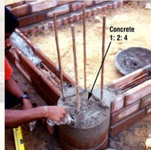
RCC Construction with Brick Cladding
