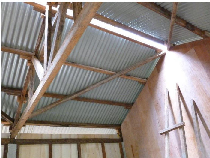
Left: Bracing has been installed below the roof, in the plane of the roof sheeting. PRCS/IFRC Haiyan Core Shelter Programme, Tabontabon, Leyte. (Photo: R. Dodds)
