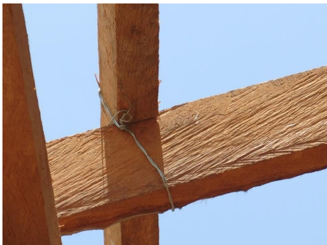
Left: The timber roofing batten has been tied-down to the timber rafter with galvanised tie wire. Credit: LandsAid housing project, San Remigio, Cebu. (Photo: W. Lechner).
