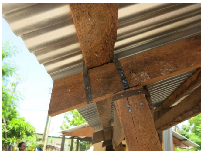
Left: The timber roofing purlins are tied down to the rafters of this shelter using salvaged pieces of steel strapping. Credit: YPDR/PAH Phase 3 housing project, Bantayan Island, Cebu. (Photo: R. Dodds)
