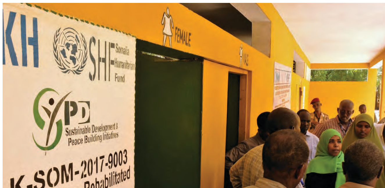
Rehabilitation of VIP latrines in Belet Weyne regional hospital (Hiraan), funded by the SHF and implemented by Diakonie Katastrophen Hilfe (DKH) and local NGO Sustainable Development & Peace Building Initiatives (SYPD). Photo: UNOCHA/Matija Kovac
