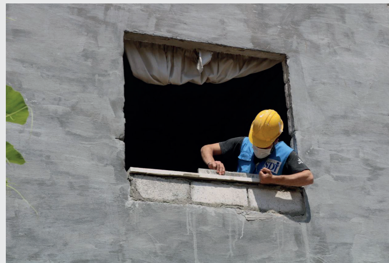
Photo Credit: SDI, shelter rehabilitation activity
