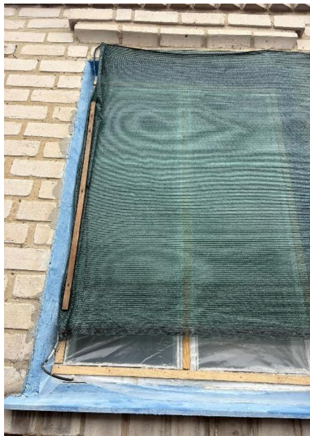
Pic. 6: A recipient of 2MT of briquettes uses plastic sheeting and mesh to cover their windows to improve insulation of their private house.
