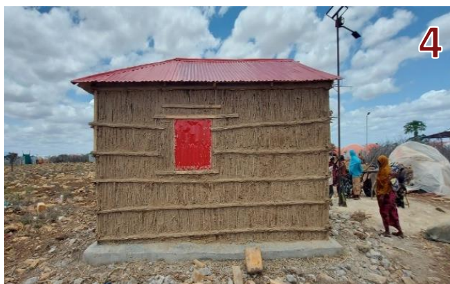
"Barako 5mx4m" type shelter with verandah made up of natural wooden stick walls plastered with mix of mud and cow dung.
