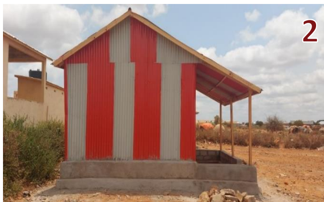
Hybrid shelter/room 4mx4m- (Block walls up to 40cm high and the rest of CGI sheets) with verandah.
