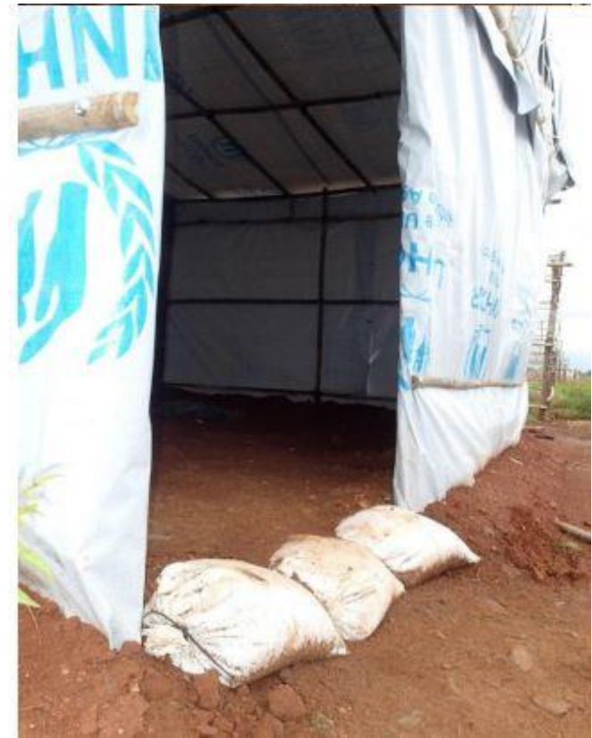
Wall base & fixing, NRC design 2014
