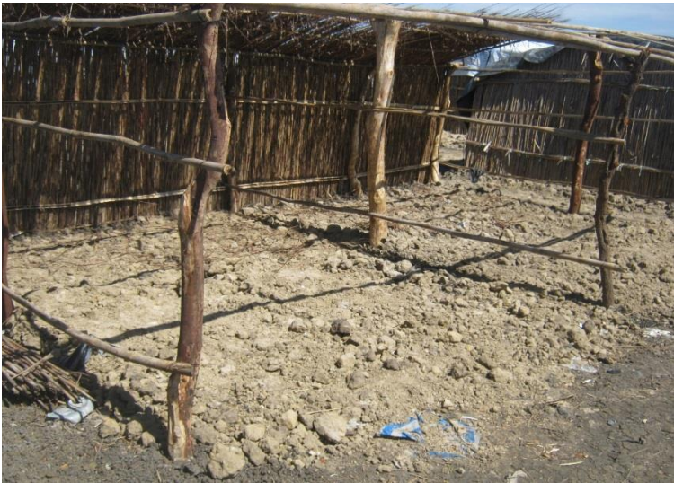
Sand backfilling , Concern design 2014
