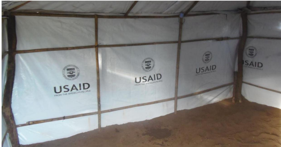
Wall structure, NRC Minkaman, 2014
