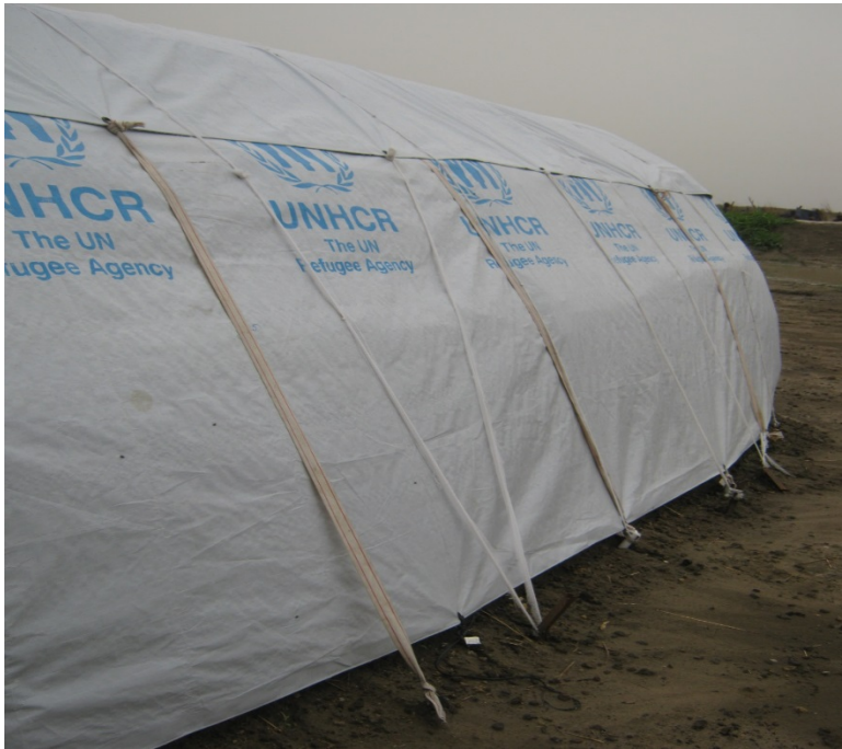
Pegging/Tying, Concern design 2014
