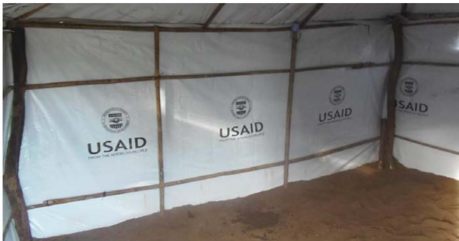
Wall structure, NRC Minkaman, 2014
