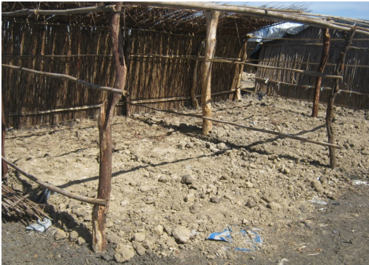
Sand backfilling , Concern design 2014
