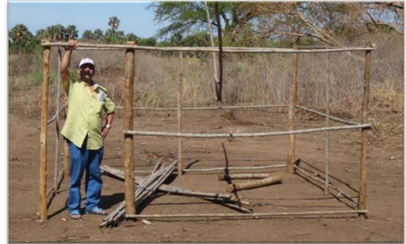
Door Frame reinforced, CRS design 2014
