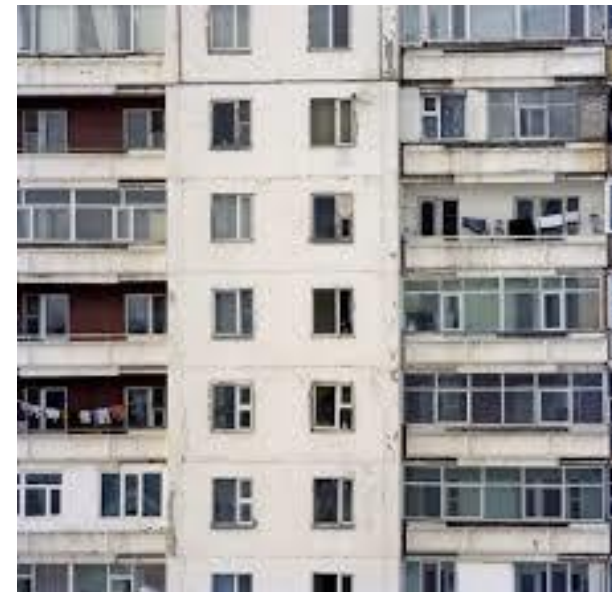
6 months rental support to move into repaired building
