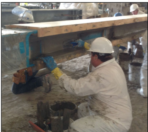
FINISH PYROCRETE WITH USE OF FORM GUIDES
