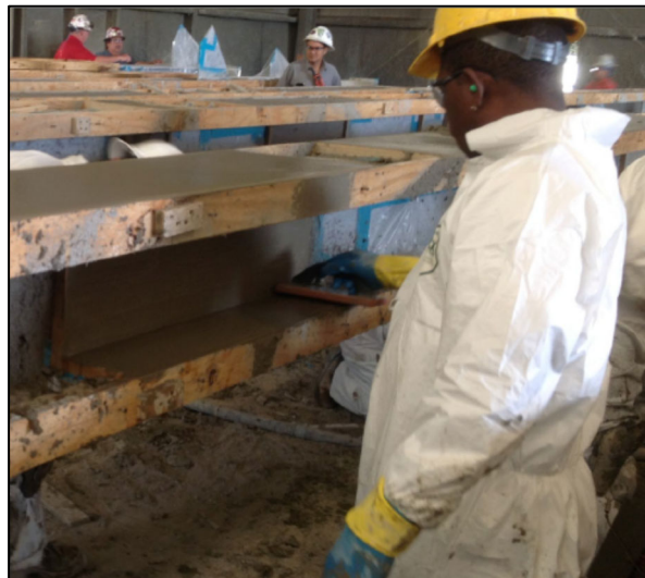
APPLIED PYROCRETE FINISHED WITH A TROWEL
