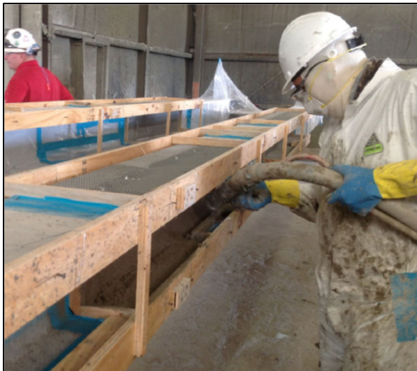
PYROCRETE SPRAY APPLIED TO REQUIRED THICKNESS
