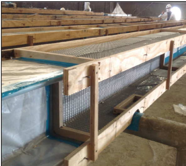
FORMS SET TO REQUIRED THICKNESS
