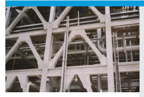
Pyrocrete 40 is designed for the fire protection of exterior structural steel, vessel skirts, and for upgrading the fire resistance of any existing concrete. Pyrocrete 40 has highly competitive ratings for UL 1709, ASTM E119 and BS-476 (hydrocarbon curve) fire standards.
