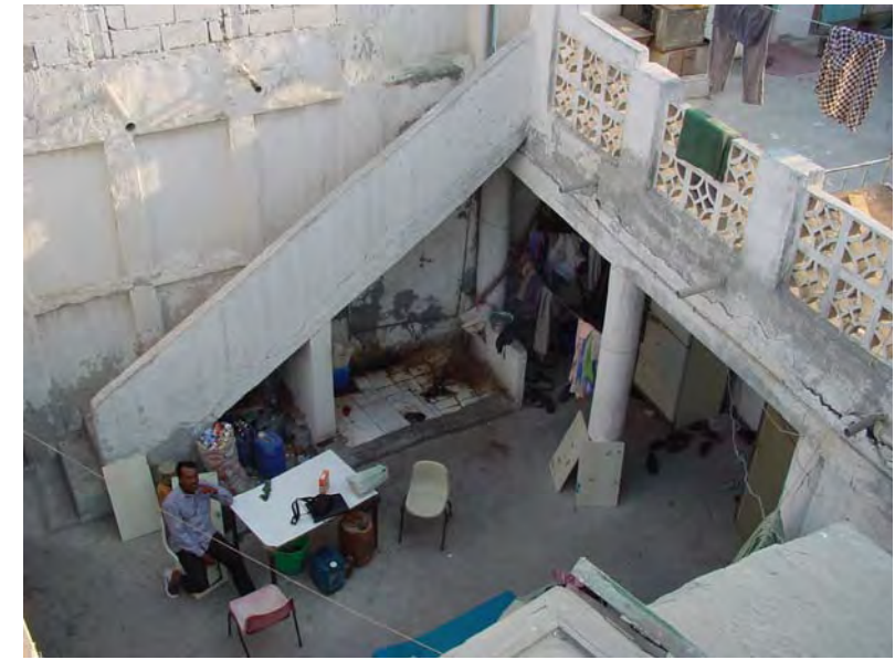
Figure 3-6: House Before Renovation
