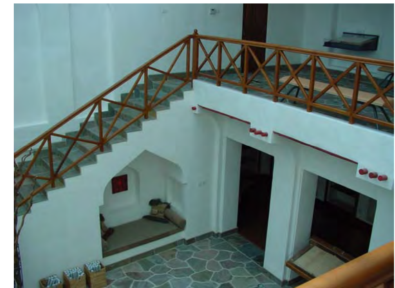
Figure 3-7: House After Renovation
