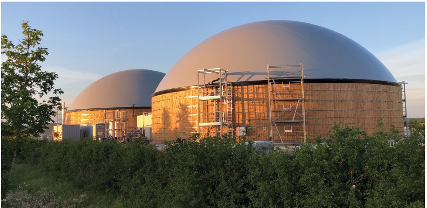
View of the digester
