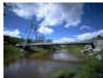
An asymmetric cable stay from a 30-metre steel tower on the right bank.
