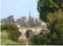
Built 1774 but completely rebuilt to lower the steep gradient in 1927.
